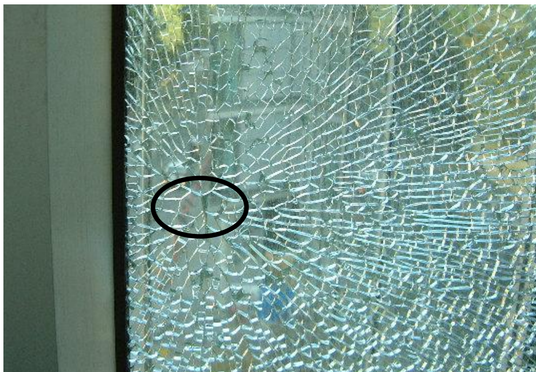
Typical breakage starting from a NiS inclusion
